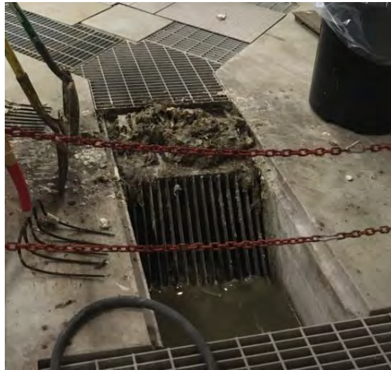
Figure 5-5: Manually Cleaned Bar Rack
