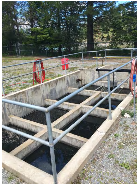
Figure 5-12: Chlorine Contact Basin
