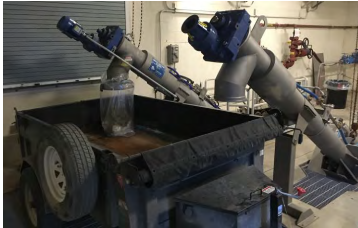
Figure 5-7: Screenings Washer Compactor
