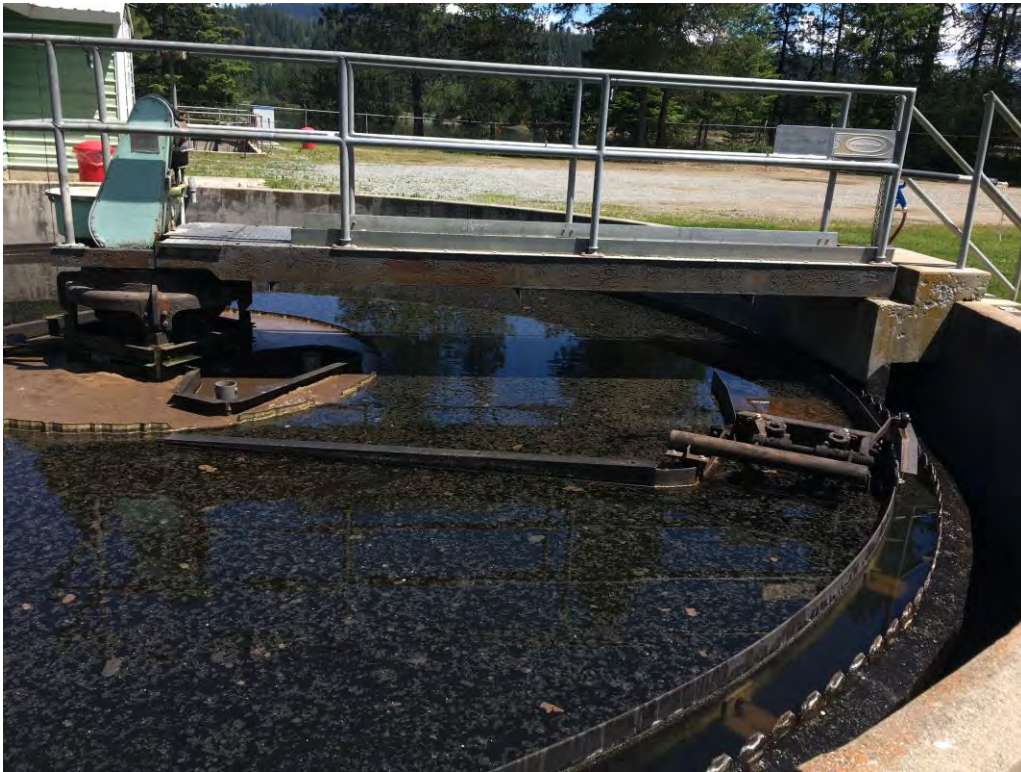
Figure 5-11: Secondary Clarifier
