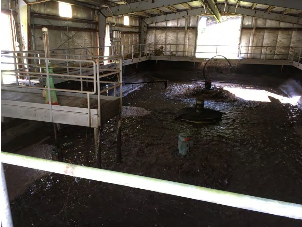
Figure 5-15: Aerobic Digester and Steel Building Enclosure
