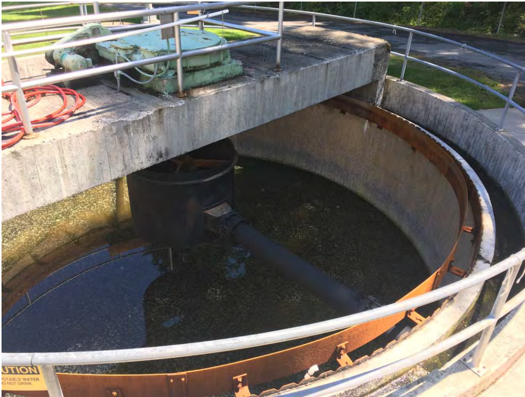
Figure 5-9: Primary Clarifier (Not Operational)
