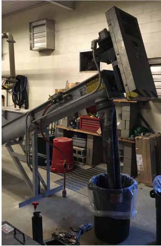
Figure 5-8: Grit Washer Conveyor
